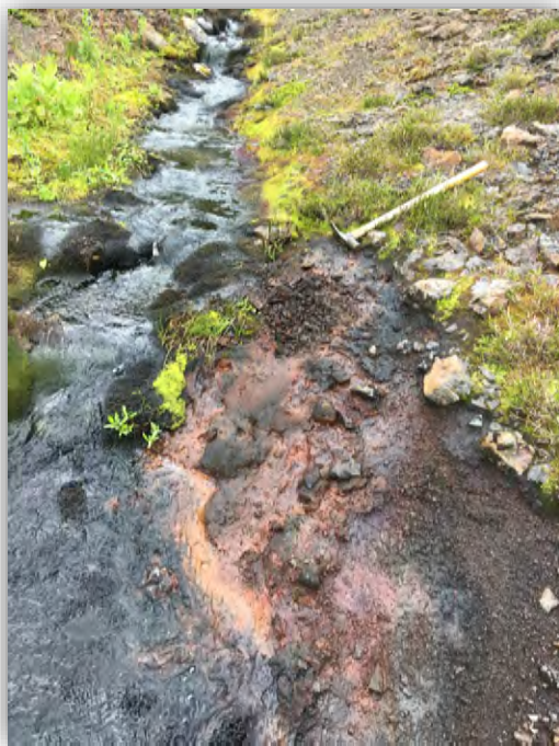
Ferrocrete Exposed in Drainage
